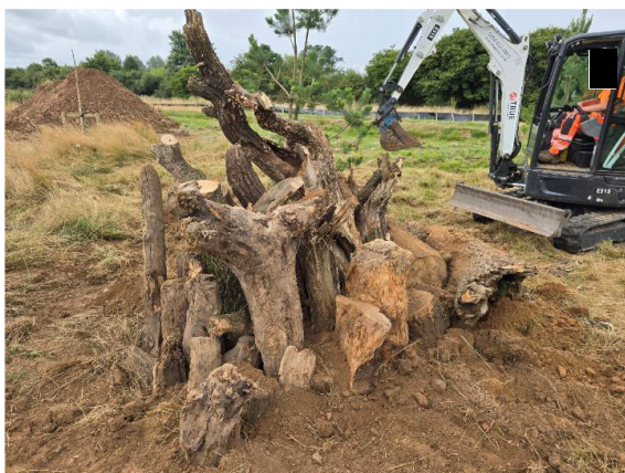
Image 22: Vertical log piles
